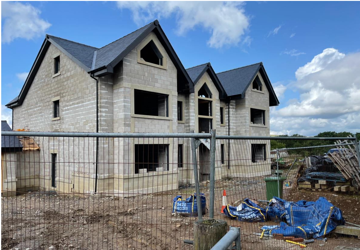
Case Officer Site photographs of application site as at 9 th August 2021:
